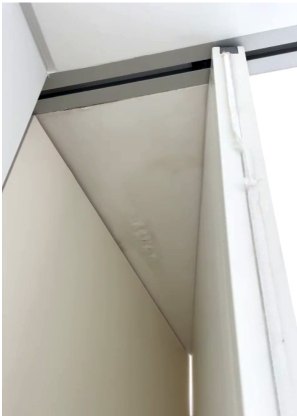
Bulged sliding doors in the kitchen.
