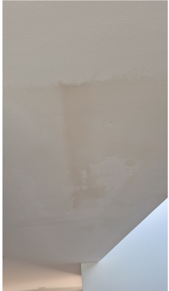
Stains on the corridor ceiling.
