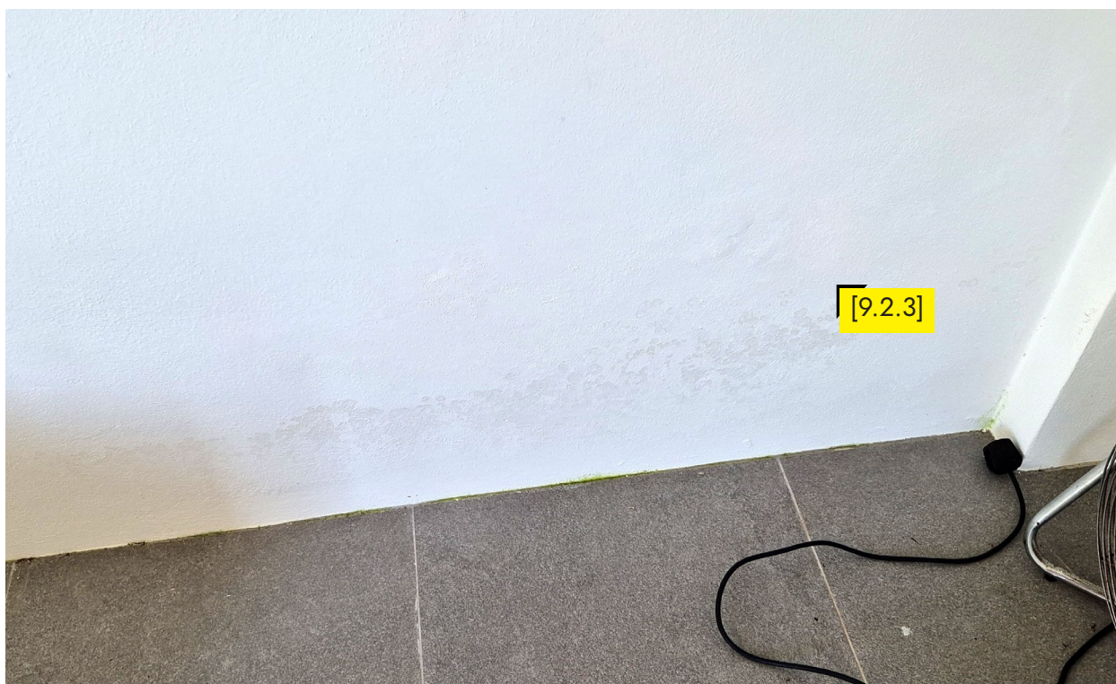
9.2.3. Crumbling plaster, soggy paint coming off.
